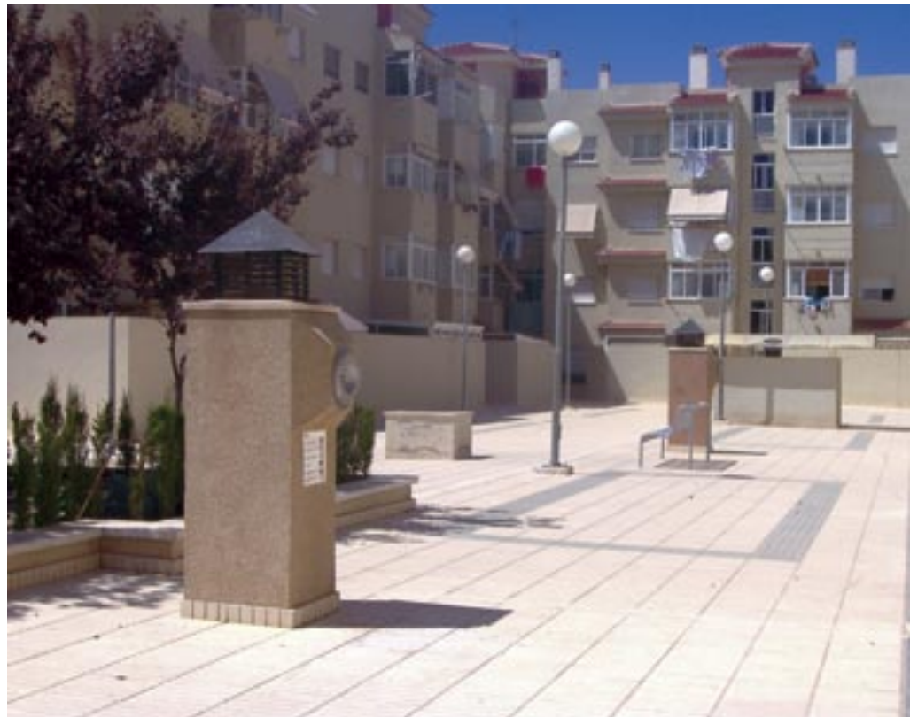
The designs of the waste inlets vary depending on the surroundings, but they are all linked to the same underground Envac system.
