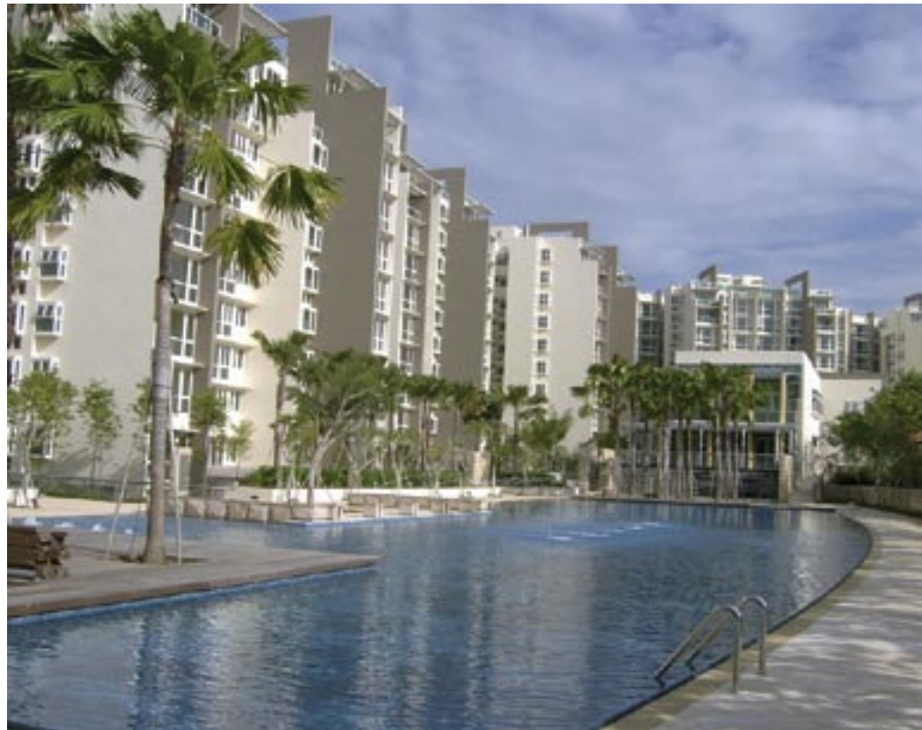
Changi Rise, Singapore - a residential district with an Envac system
