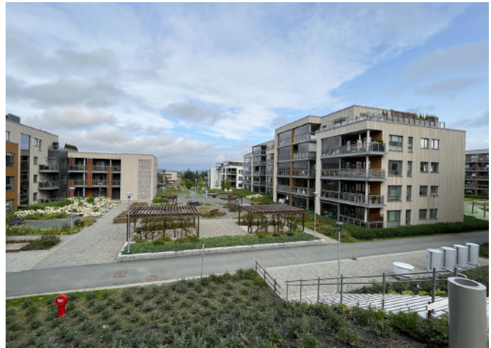
Ladebyhagen apartments connected to Envac terminal in the area that eliminates heavy garbage truck movement.
