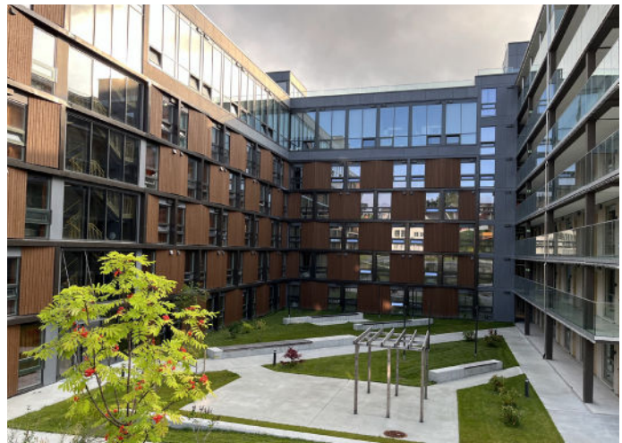
Illustration of Campus Nardo, student housing new project in Trondheim city using the Envac automatic waste collection solution.
