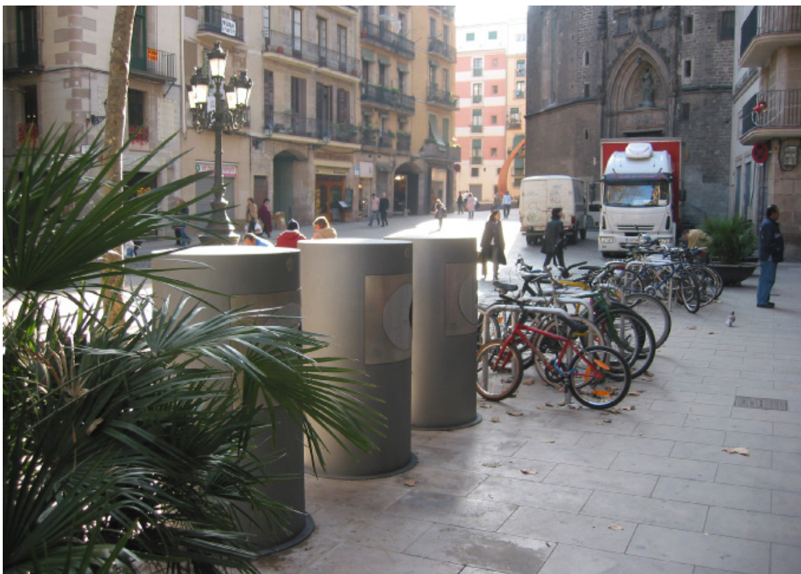
Pneumatic waste inlets in Barcelona, where the municipality owns the facility financed through a local tax.
